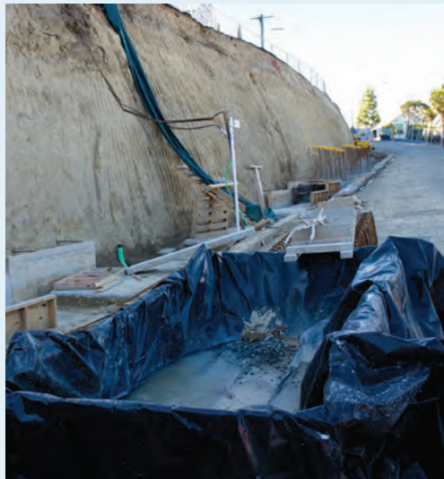
A contained concrete wash-off.
