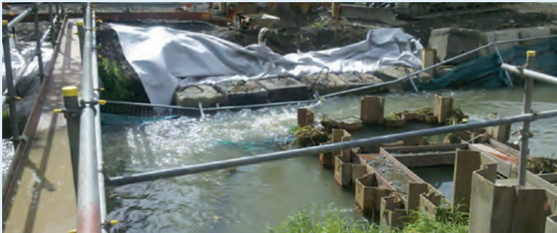
Cofferdams and stabilised riverbanks.
