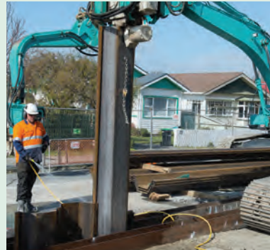
A sheet-piling installation.
