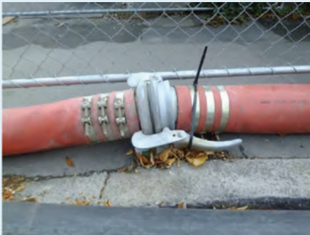
Couplings for added security on a discharge pipe. Float alarms in a manhole.
