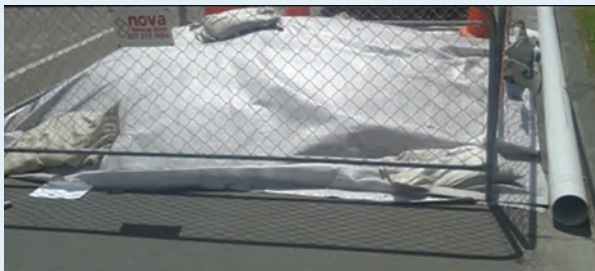
Covered stockpile with kerb diversion pipe.
