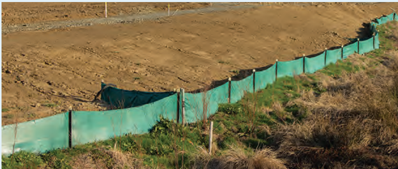
A silt fence installed along land contours.
