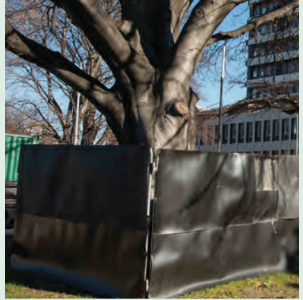
Protective fencing for a tree on a work site.
