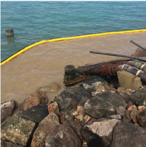
A sediment curtain with floating booms.
