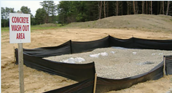
A concrete washout area.
