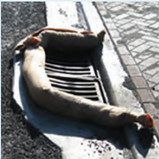
A catch-pit protection.
