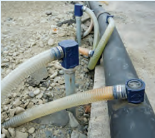
Well points are installed for dewatering.
