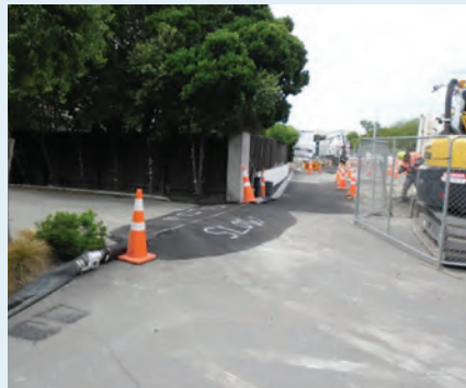
Security to prevent vandalism. Access ramps to prevent pipe damage.
