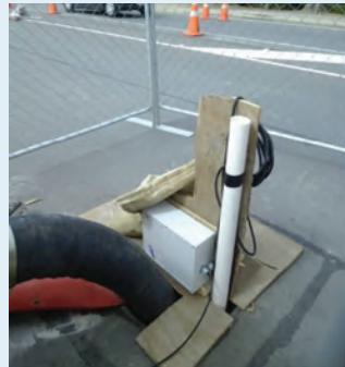
Couplings for added security on a discharge pipe. Float alarms in a manhole.
