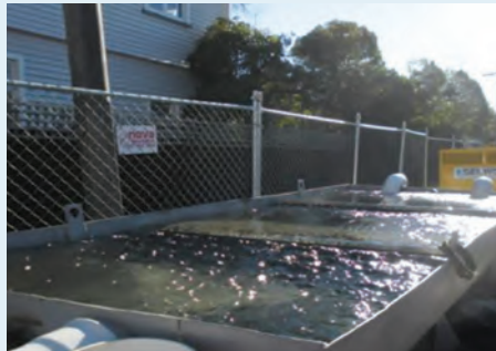
A dewatering tank with baffles.
