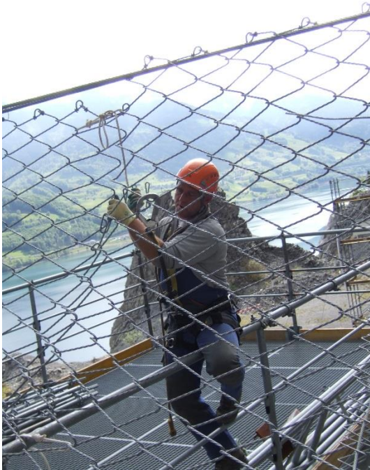
c) Unscrew the outermost spiral
