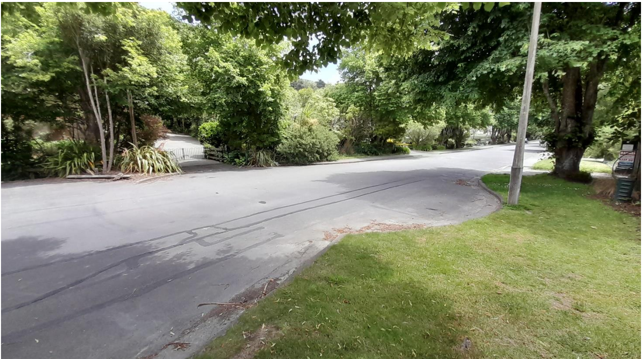
Photograph 2-2: Existing Turning Head at 114 Bowenvale Avenue
