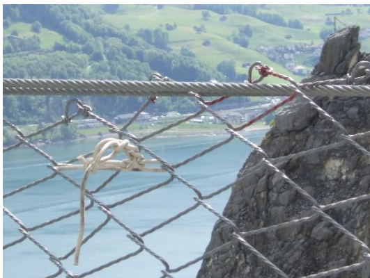
a) Relieve the strain on the outermost spiral of the damaged area
