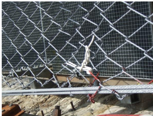
a) Relieve the strain on the outermost spiral of the damaged area
