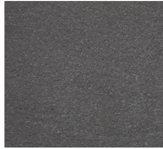
Asphalt (Carriageway/ footpath)
