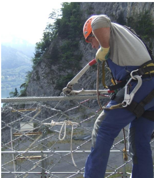
b) Cut open the eyelet connection of the outermost spiral
