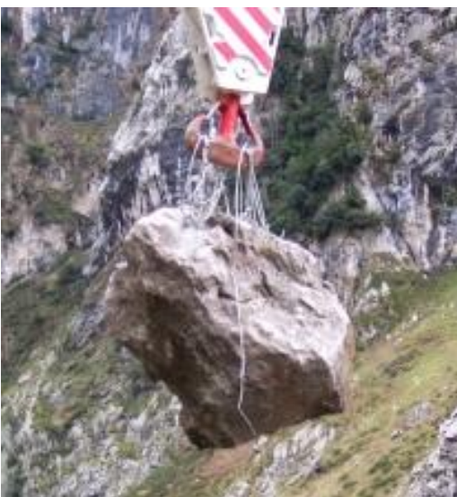
Lifting the block out with the aid of a crane
