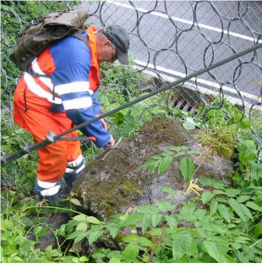
Breaking a block down using explosives
