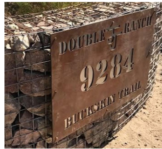
Corten Entrance Sign (Fixed to gabion basket retieing wall)
