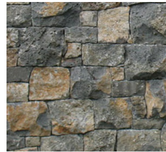
Split face basalt columns (Bridge entrance)
