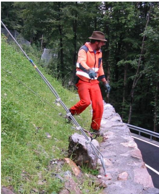
Lowering stones safely (secured with a rope)
