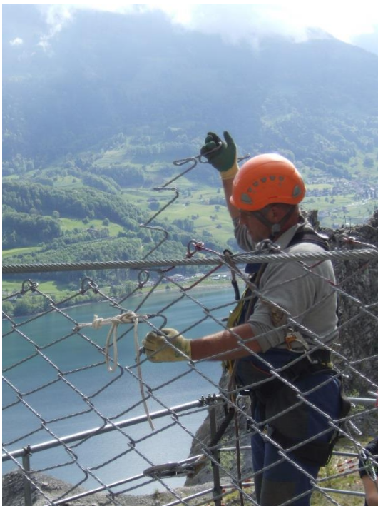
f) Connect the new net to the intact adjacent nets with a spiral (or with shackles).
