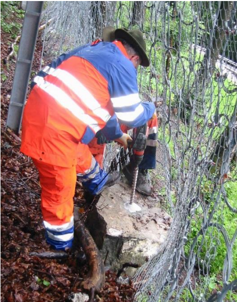
Fitting the block with haulage hooks
