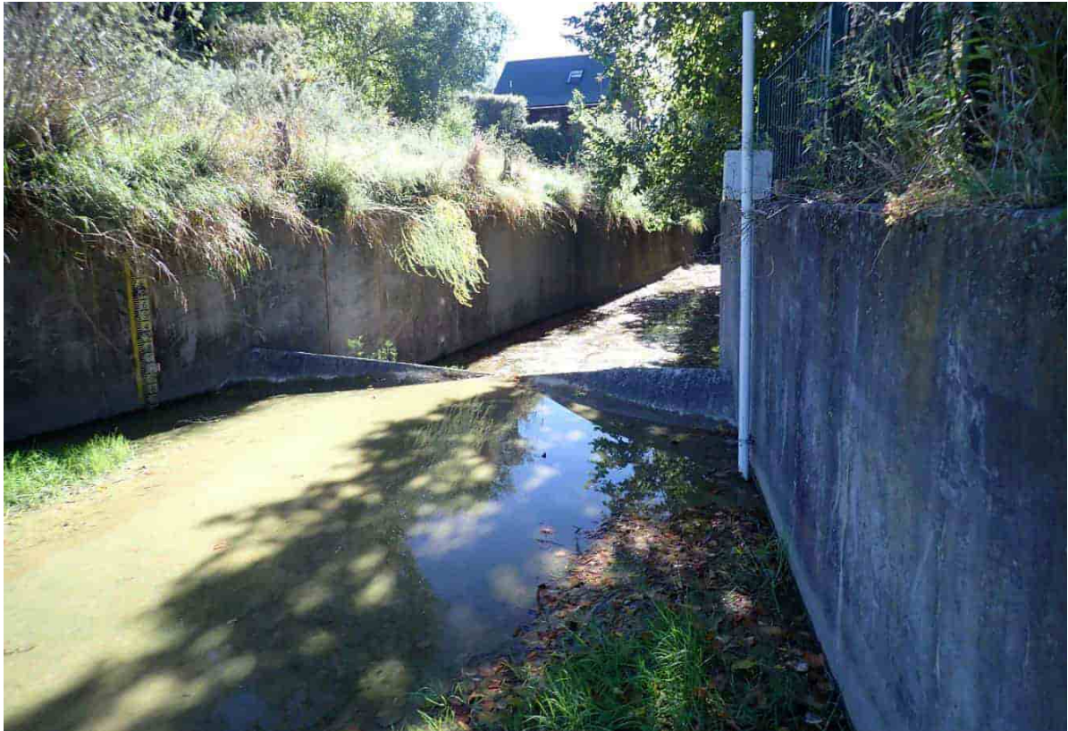
Figure viii. Looking downstream at Bowenvale Stream, downstream of the existing CCC flood control area. This waterway is concrete-lined to the Heathcote River, with no visible fish baffles.
