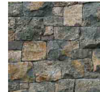
Split face basalt columns (Bridge entrance)
