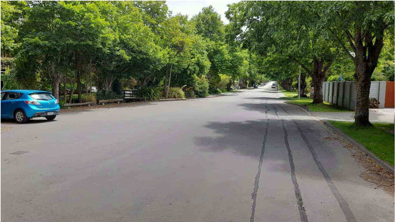
Photograph 2-1: Bowenvale Avenue Looking North at Proposed Intersection Location
