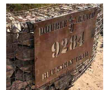
Corten Entrance Sign (Fixed to gabion basket retaining wall)
