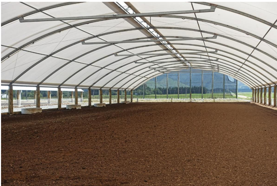
Photo 16. A North Island hoop structure in a windy site.
