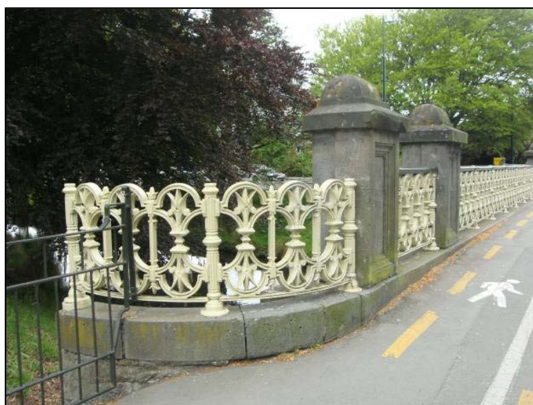
Figure 1.15. Cast iron balustrade on Armagh Street Bridge. Source: DPAL, 2012
