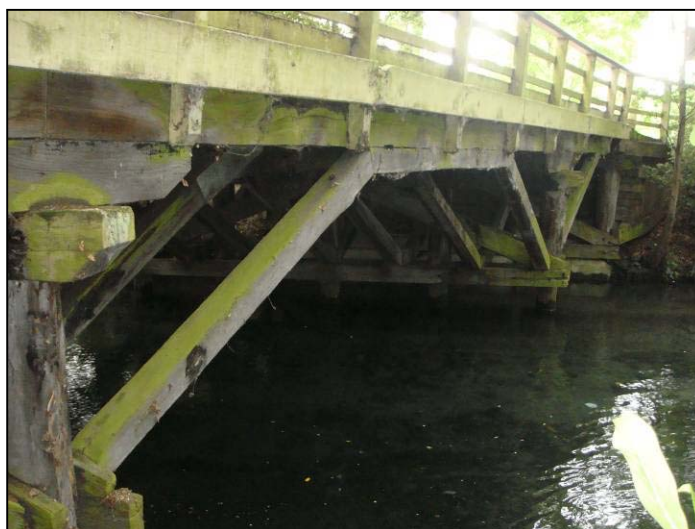
Figure 1.25. Timber elements supporting the bridge. Source: DPAL, 2012
