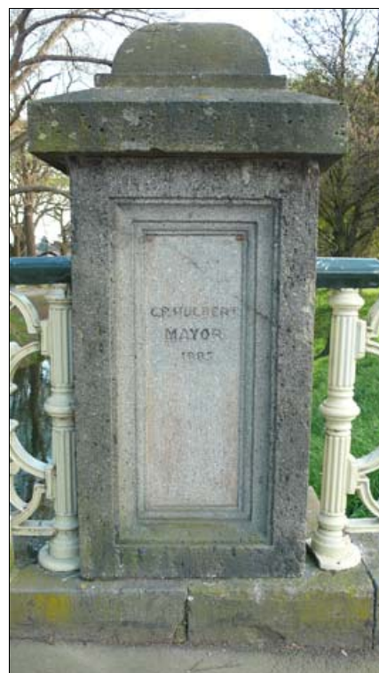
Figure 1.22. Diagonal cracking through abutment. Source: L. Beaumont, 2011
