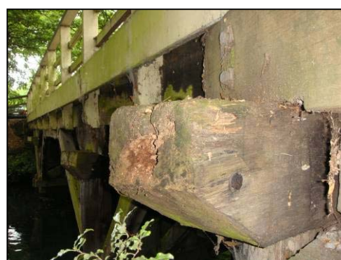
Figure 1.27. General deterioration and movement of handrail (left) and general decay in timber (right).
