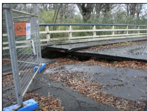
Figure 1.26. Subsidence of abutment beside road.
