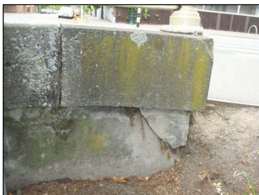
Figure 1.20. Cracked footing (left) and rust on the balustrade (right).
