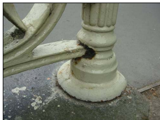
Figure 1.20. Cracked footing (left) and rust on the balustrade (right).
