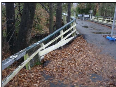
Figure 1.27. General deterioration and movement of handrail (left) and general decay in timber (right).
