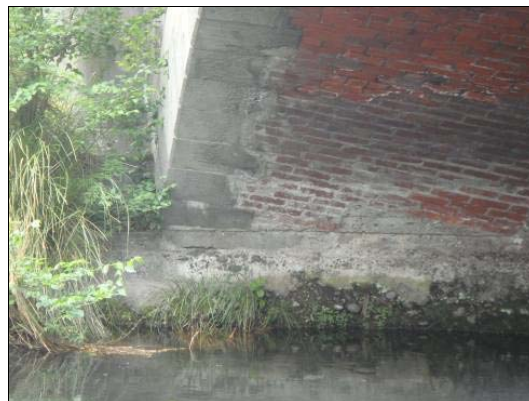
Figure 1.19. (Left) Erosion of plaster on bridge face and (right) signs of efflorescence on brick arch
