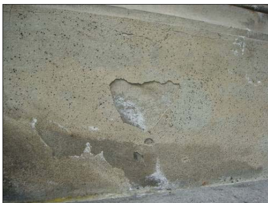
Figure 1.19. (Left) Erosion of plaster on bridge face and (right) signs of efflorescence on brick arch
