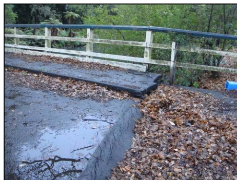
Figure 1.26. Subsidence of abutment beside road.
