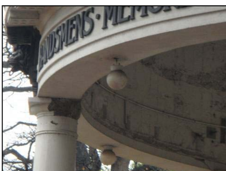
Figure 1.52. Damage to capitals with loss of plaster (left) and damage to plinth base of columns. Source: DPAL
