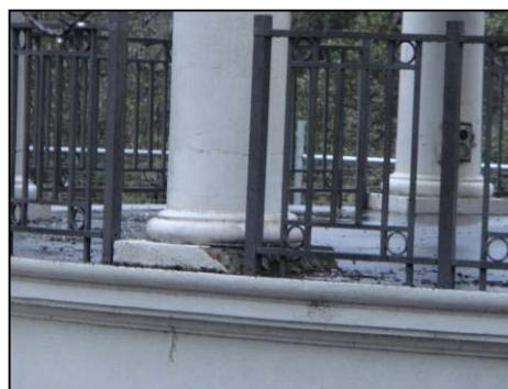
Figure 1.52. Damage to capitals with loss of plaster (left) and damage to plinth base of columns. Source: DPAL
