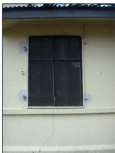
Figure 1.40. Cracks in façade (left) and erosion in the marble plaque and chipped plasterwork (right). Source: DPAL, 2012
