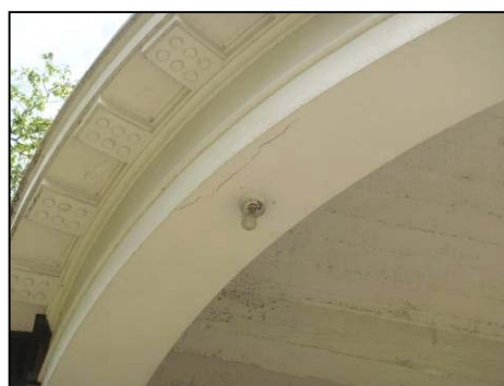
Figure 1.50. Crack in pilaster (left) and crack on underside of architrave beam (right). Source: DPAL
