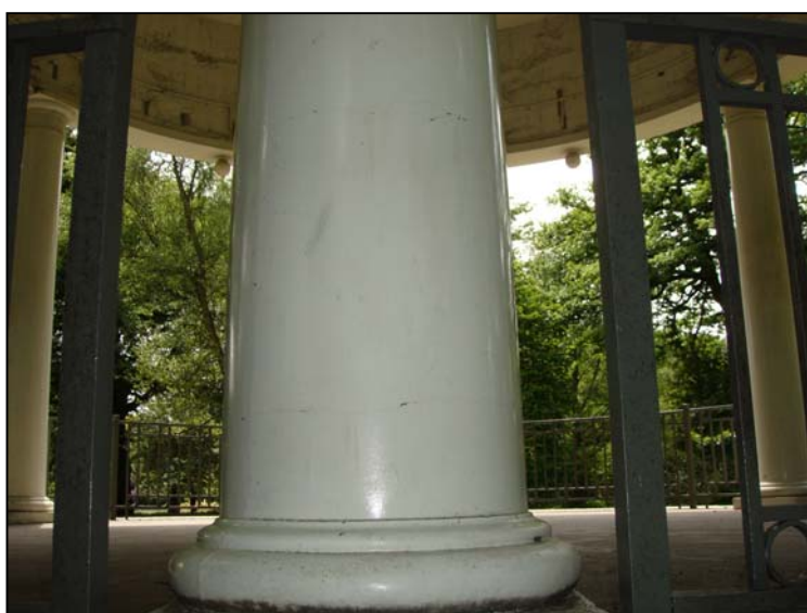
Figure 1.47. Smooth plaster finish of columns, 2012.
