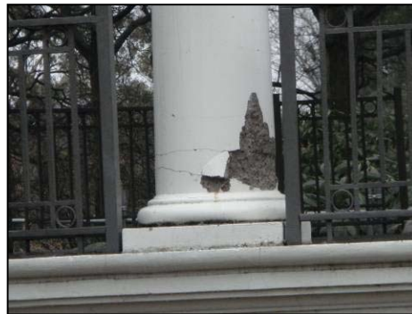
Figure 1.51. Damage to capitals (left) and horizontal cracking on columns with fallen plaster. Source: DPAL
