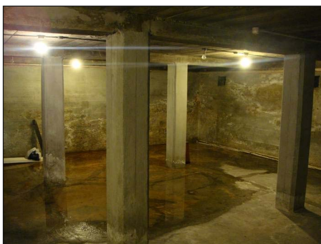
Figure 1.71. Basement with supporting reinforced concrete columns. Source: DPAL, 2012
