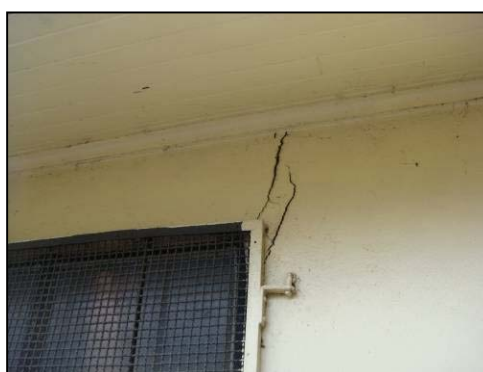
Figure 1.41. Cracks in front façade around the window to the west of the front entrance. Source DPAL, 2012
