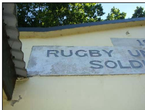
Figure 1.40. Cracks in façade (left) and erosion in the marble plaque and chipped plasterwork (right). Source: DPAL, 2012
