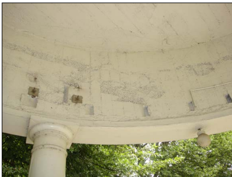
Figure 1.48. Lion head bolt fixings on inside of rotunda, 2012. Source: DPAL
