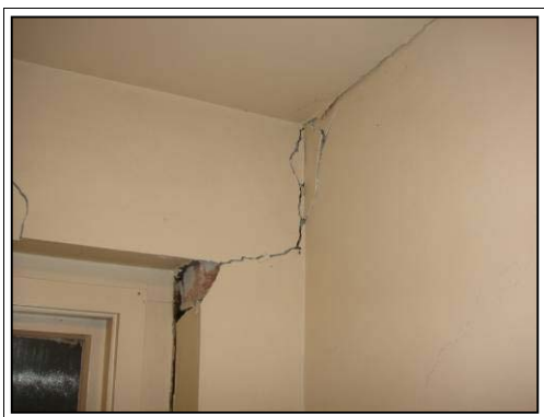
Figure 1.73. (left) Substantial cracks in outer toilet wall around the window and loss of plaster, 2012. Figure 1.74. (right) Steel bracing against the wall inside the portico entry, 2012. Source: DPAL
