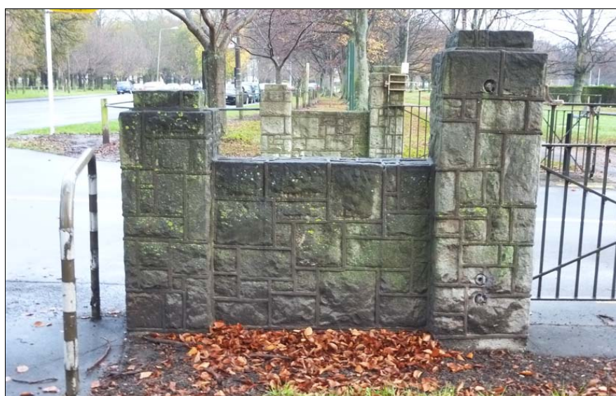
Figure 1.30. MacGibbon gates showing original fixation points to earlier fence. Source: L Beaumont, 2011
