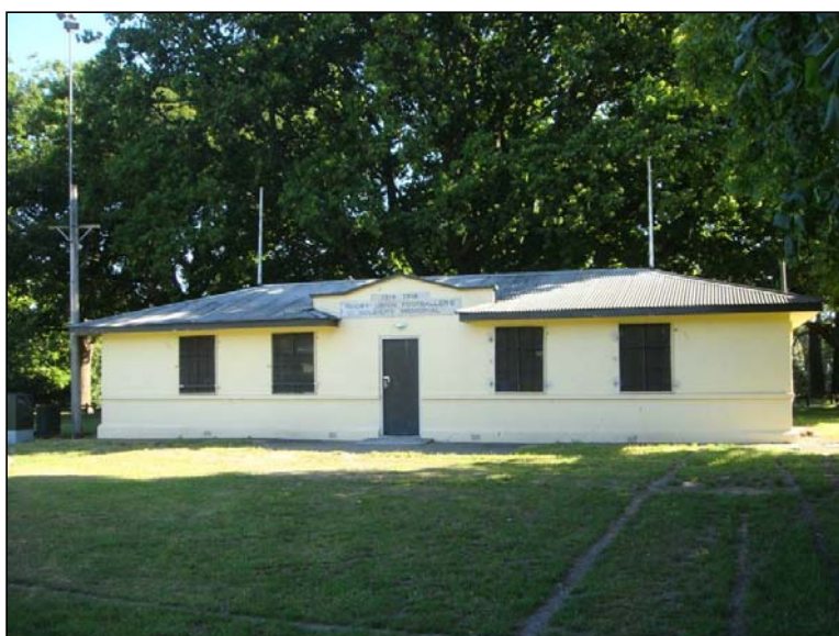
Figure 1.39. Front elevation of the Rugby Union Footballers Soldiers Memorial building. Source: DPAL, 2012
