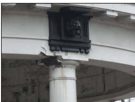
Figure 1.51. Damage to capitals (left) and horizontal cracking on columns with fallen plaster. Source: DPAL
