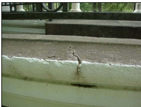
Figure 1.49. Cracks in concrete base and chipped plaster. Source: DPAL
