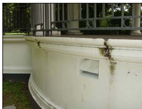
Figure 1.49. Cracks in concrete base and chipped plaster. Source: DPAL
