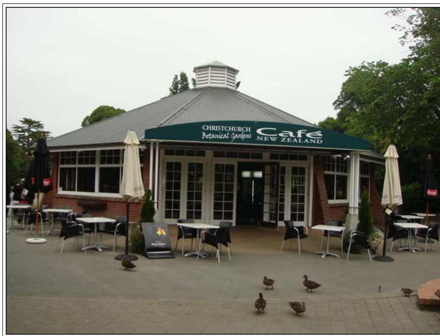
Figure 1.85. The front elevation to the café with multi-paned doors, 2011.
