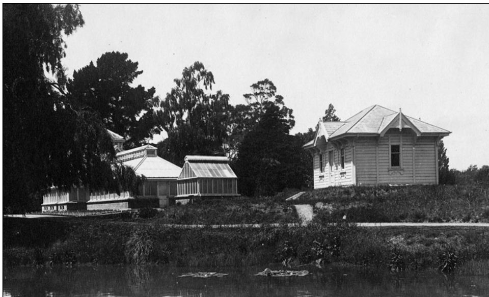
Figure 1.73. Magnetographic House, also called the Variation Observatory (right) and Orchid House (centre) Source: C722, Carnegie Institution of Washington,
