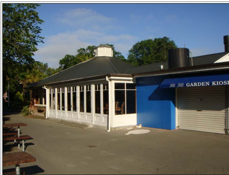
Figure 1.86. The conservatory and kiosk on the north western side of the building. Source: DPAL, 2011
