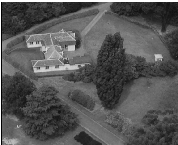
Figure 1.75. Aerial view of the Magnetic Observatory showing the extent of the operation and the setting in 1962. Source: Whites Aviation, WA-61184-F, ATL
