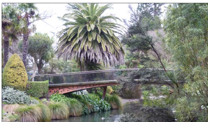
Figure 1.84 Extant bridge, now known as North Bridge, 2011 Source: L. Beaumont
