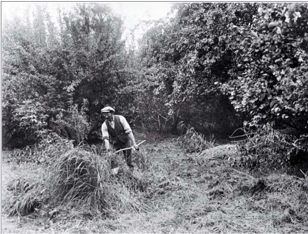
Figure 3.65. Clearing overgrown vegetation at Millbrook, 1923 Source: PhotoCD 16, IMG0083, CCL
