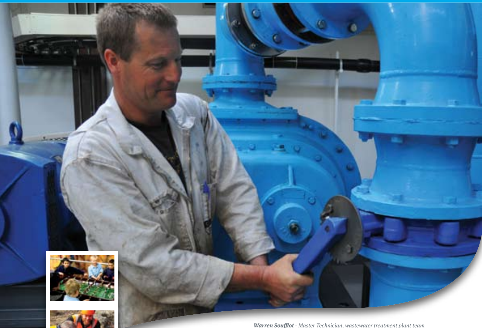
Warren Soufflot - Master Technician, wastewater treatment plant team
