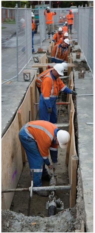
Contractors install large 66,000 volt cable between Orion's major substations in St Albans and Dallington.
