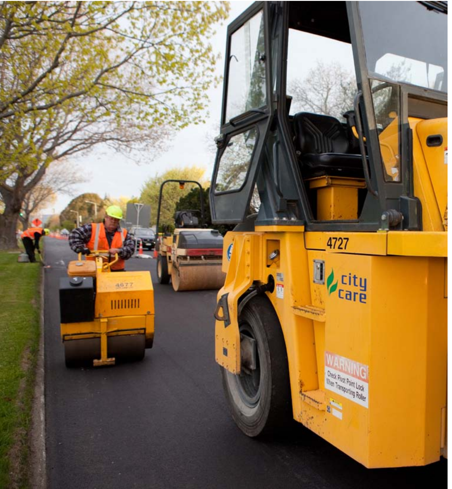
City Care workers repair roads as part of Christchurch's infrastructure rebuild.
